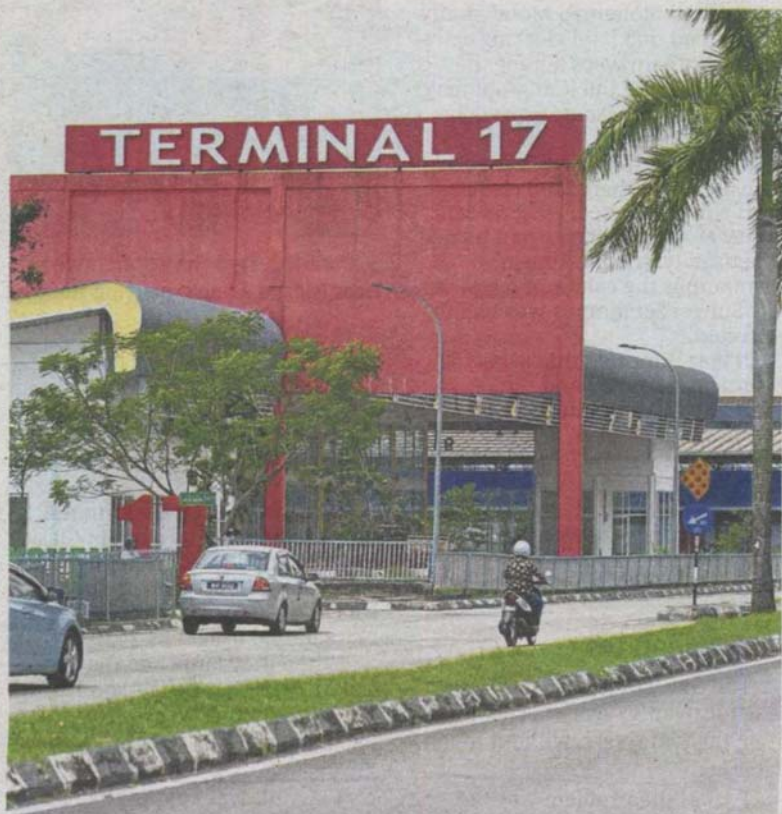
Travellers have been waiting for months for the Section 17 bus terminal to open in Shah Alam.
